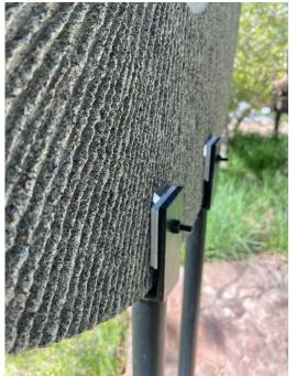
3. With help, lift your pendant/disc into place and use the provided shims to hold your pendant upright. Four (4) shims are provided, you can use two on each side or one and one, depending on the thickness of your disc.
